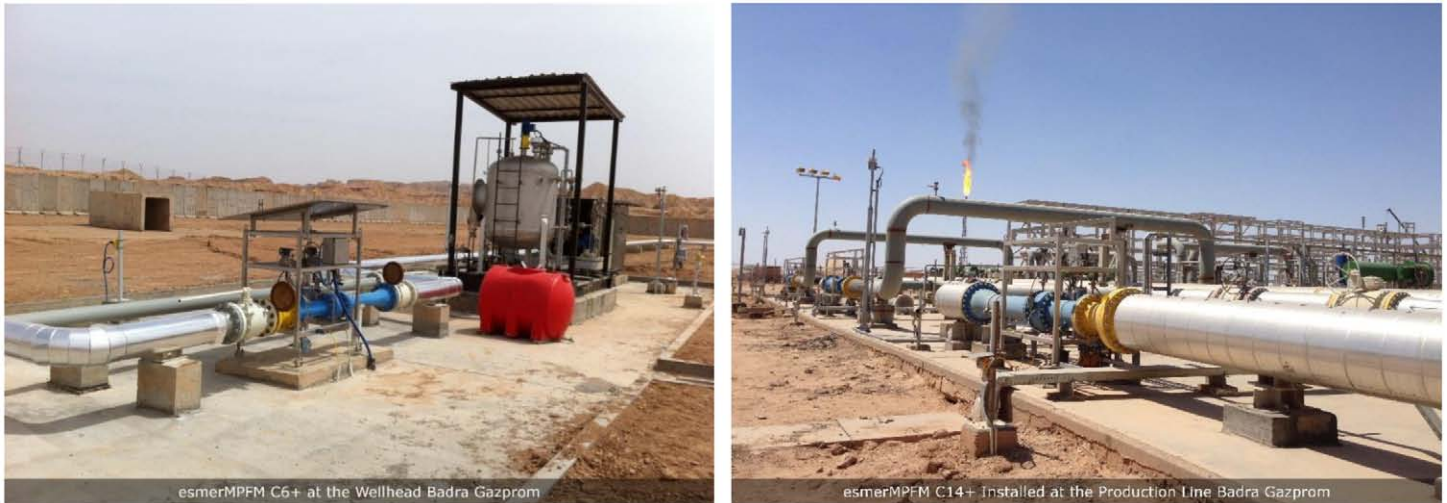
Figure 1—ESMER MPFMs at the Well Head and the Production Line at Badra Oil Field.
